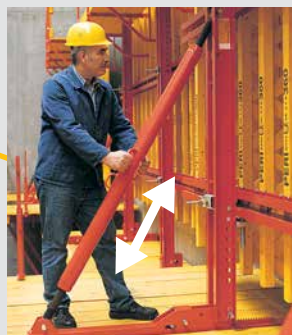
Precise adjustment of the angle of inclination With Adjustable Brace CB 164-224.
