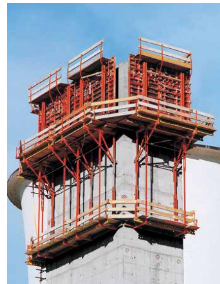
Administration building CB 240 with finishing platform and TRIO.
