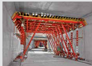
Tunnel Formwork
