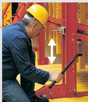
Element height adjustment For VARIO GT 24. With Height Adjusting Unit CB.
