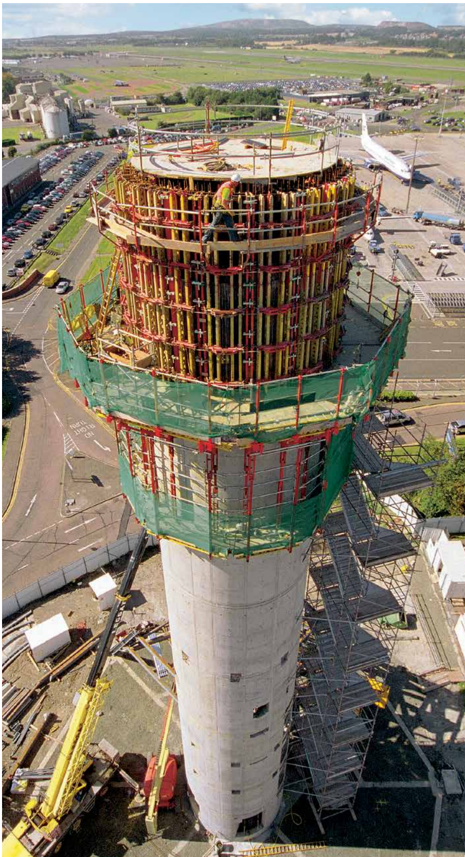
Airport control tower 46 m high, external Ø 6.85 m. With PERI RUNDFLEX and CB 240 brackets.
