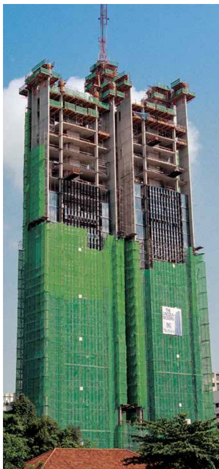
30-storey apartment building CB 240 and CB 160 scaffold brackets with VARIO GT 24.
