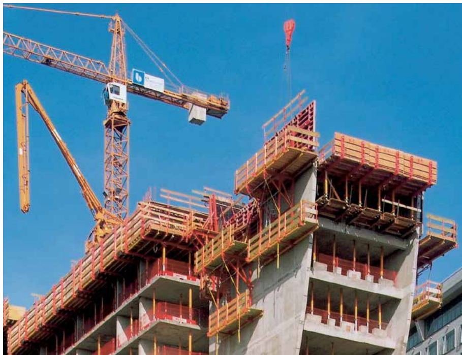
Hotel construction CB 240 scaffold brackets complete with finishing platform and TRIO.
