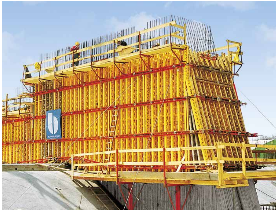
Rear side of the weir pier. The VARIO GT 24 could be easily adapted to suit the inclined rear wall requirements.
