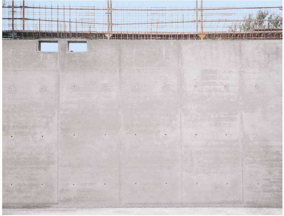
An orderly pattern of ties spaced at 0.75 x 1.18 m and smooth, architectural concrete are the result (Secondary School in Kletov).
