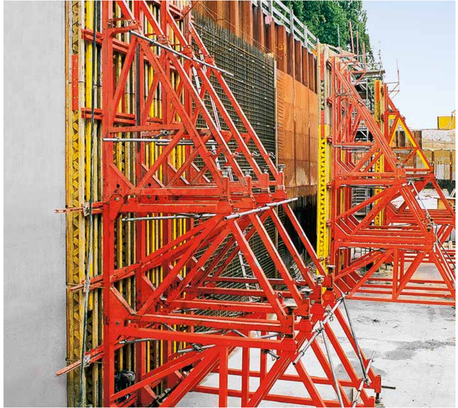
Max. concreting height of 8.75 m, Brace Frame SB-A0, A, B and C with VARIO GT 24 wall formwork.
